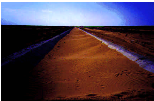
Photo: eg24-30a: New irrigation canal under construction through mined areas. The government wants to release land here for irrigated crops, using underground water. Note the blown sand indicating that sand is very mobile here under the right conditions.
